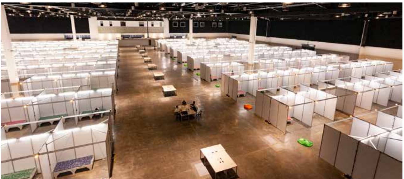
Makati Development Corporation converted the exhibition halls of the World Trade Center Manila into the 500-bed We Heal as One Center within 7 days.
