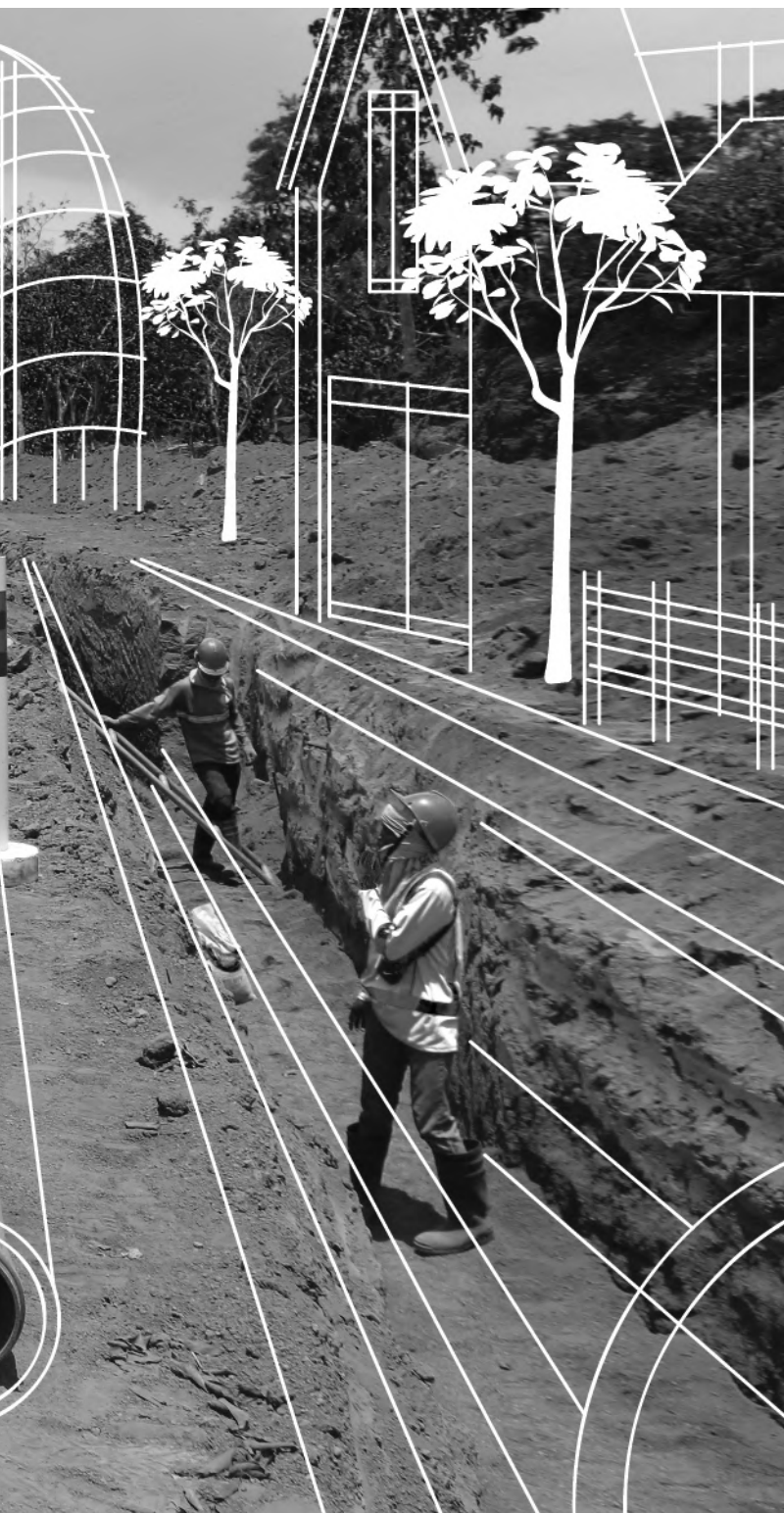
Pipelaying in Laguna Technopark
