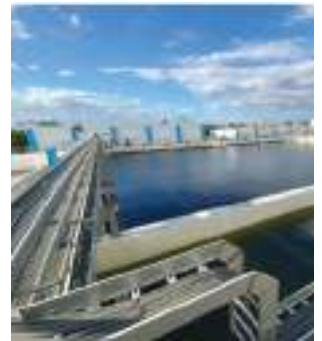
Sewage Treatment Plant at Ilugin, Pasig City
