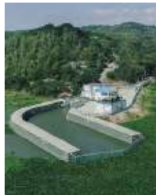
Raw water intake at Cardona, Rizal
