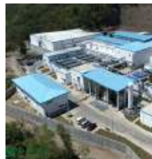
Water treatment plant at Cardona, Rizal
